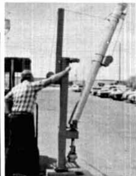
Tilting the tower over is a one-man task with the Wilson bases. (Shown above is the RB-61A. Rotor is not included.)
